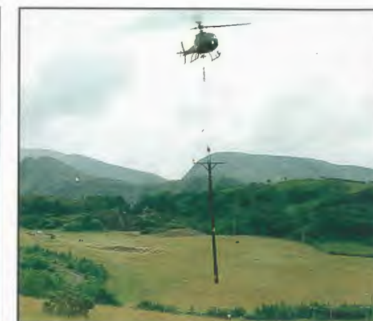
Far left, the helicopter lifts up an overhead line wooden pole; left, the pole is transported over the rugged Snowdonia terrain; and, above, the pole is lowered into position.
